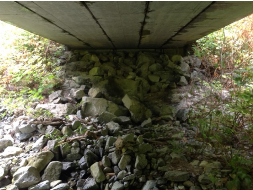
Left Bank Abutment when facing downstream
