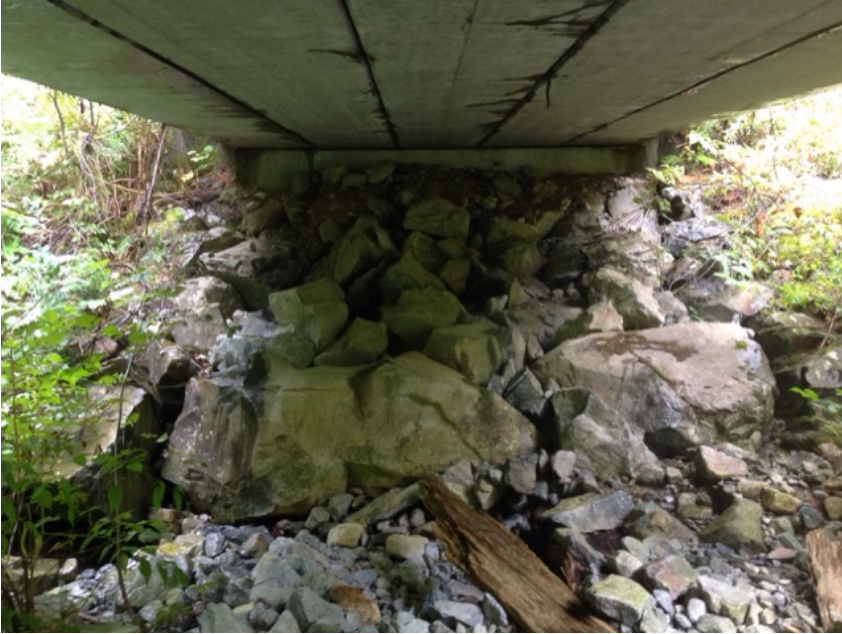
Right Bank Abutment when facing downstream
